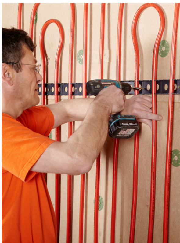
Fastening a hydronic heat element
