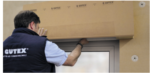
Installing the housing after insulation board installation
