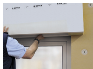
Installing the housing after installation of the insulation boards
