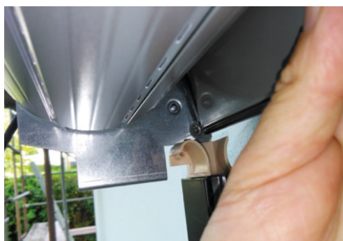
Feeding the sunshade into the tracks
