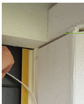
Flush interior housing ends
